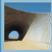
Corrugated Steel Culverts
